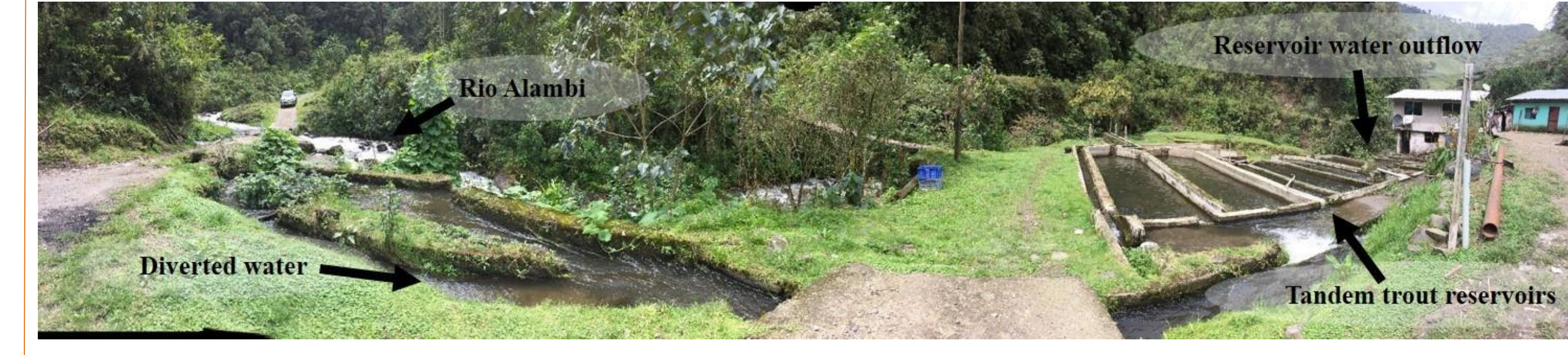
Figure 3. General flow-through design of trout farms in the region.
